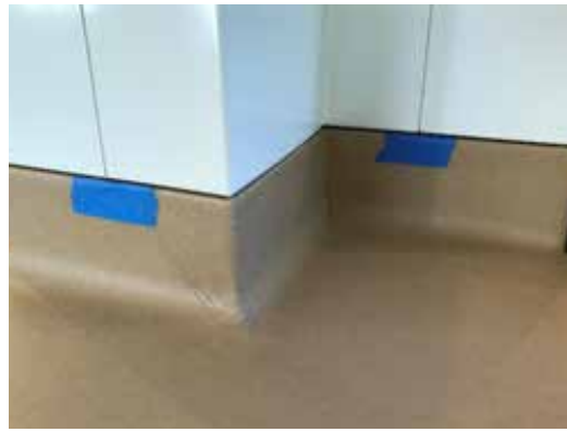
8. When heat welding the walls, place several layers of tape to prevent burning the floor. Once welded, trim any excess.
