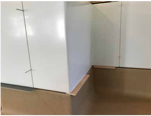
7. Use 2d or 3d nails, to space between panels, for heat welding and expansion.
