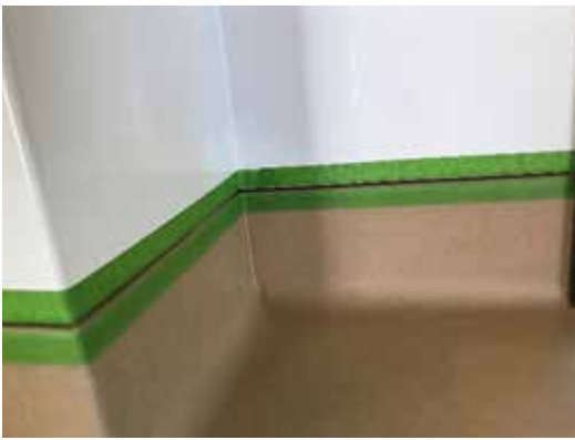
9. Tape off the rebate and apply tamper-resistant security sealant.
