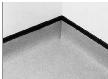
6. Heat weld to complete the section. See Heat welding on page 36 for more info about heat welding.
