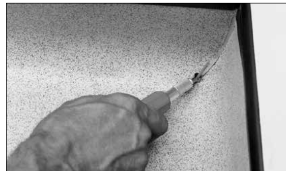
2. The X-ACTO small round router blade should be used for trimming the cooled weldrod on internal corners.
