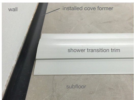
1. After subfloor preparation, cut shower transition trim to desired length.
