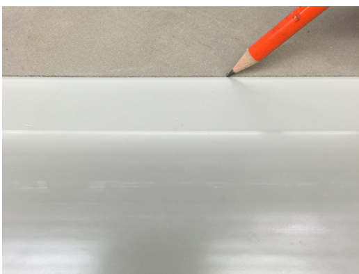
4. Mark location where shower transition trim will be installed with pencil.
