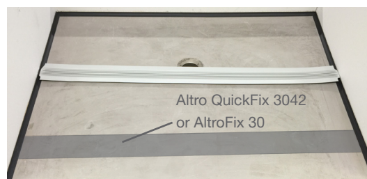
5. Apply Altro QuickFix 3042 adhesive within the pencil lines and onto the cove former. Alternatively, Altrofix 30 adhesive can be used, however the fast setting QuickFix adhesive is preferred.
