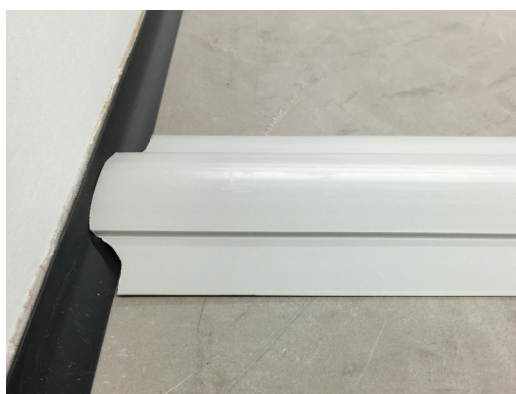
2. Cut shower transition trim, as shown above, to fit installed cove former.
