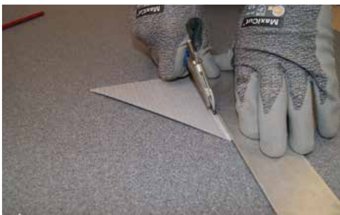
3. Groove the back of material out approximately 1/3rd depth at the point where the pad out section will be on the corner of the wall.
