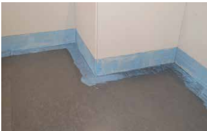
1. Apply adhesive to the floor and wall where material is to be covered.
