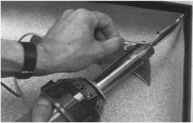
1. Groove the lower section of the joint, but not the upper
